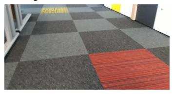
Greenstream were appointed to replace existing carpets – which were in poor condition after long-term extended use – for recycling and re-use. Across all three phases, a total floorspace of 1,213m² was carpeted. Re-used carpet tiles accounted for 530m², equivalent to 44% of the total floorspace.
